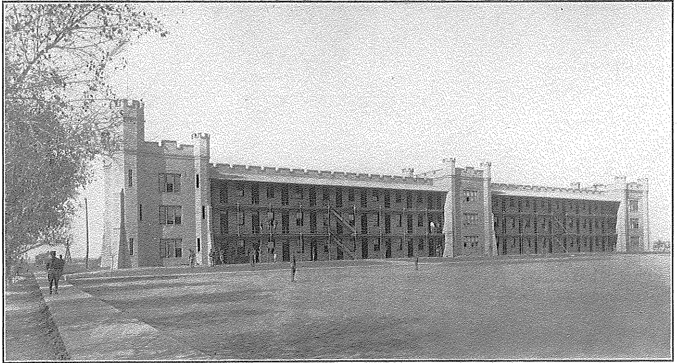
FRONT VIEW OF HAGERMAN BARRACKS
